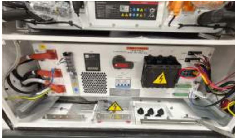
Figure 5-17 Position of Network Port
