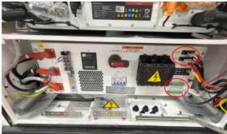
Figure 5-18 Position of CONN1–CONN4 Terminals
