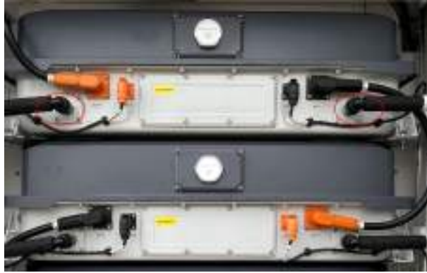
Figure 5-14 Positions of Liquid Cooling Pipe Fittings
