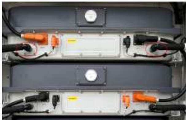
Figure 5-7 Positions of Liquid Cooling Pipes
