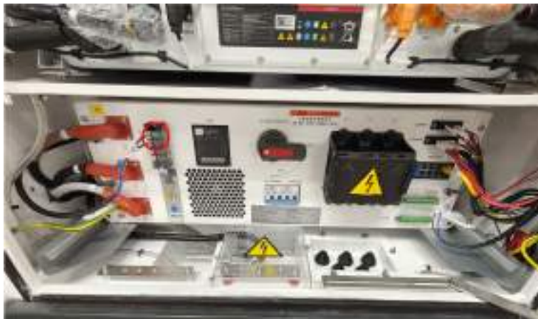
Figure 5-16 Position of Power Supply Cable
